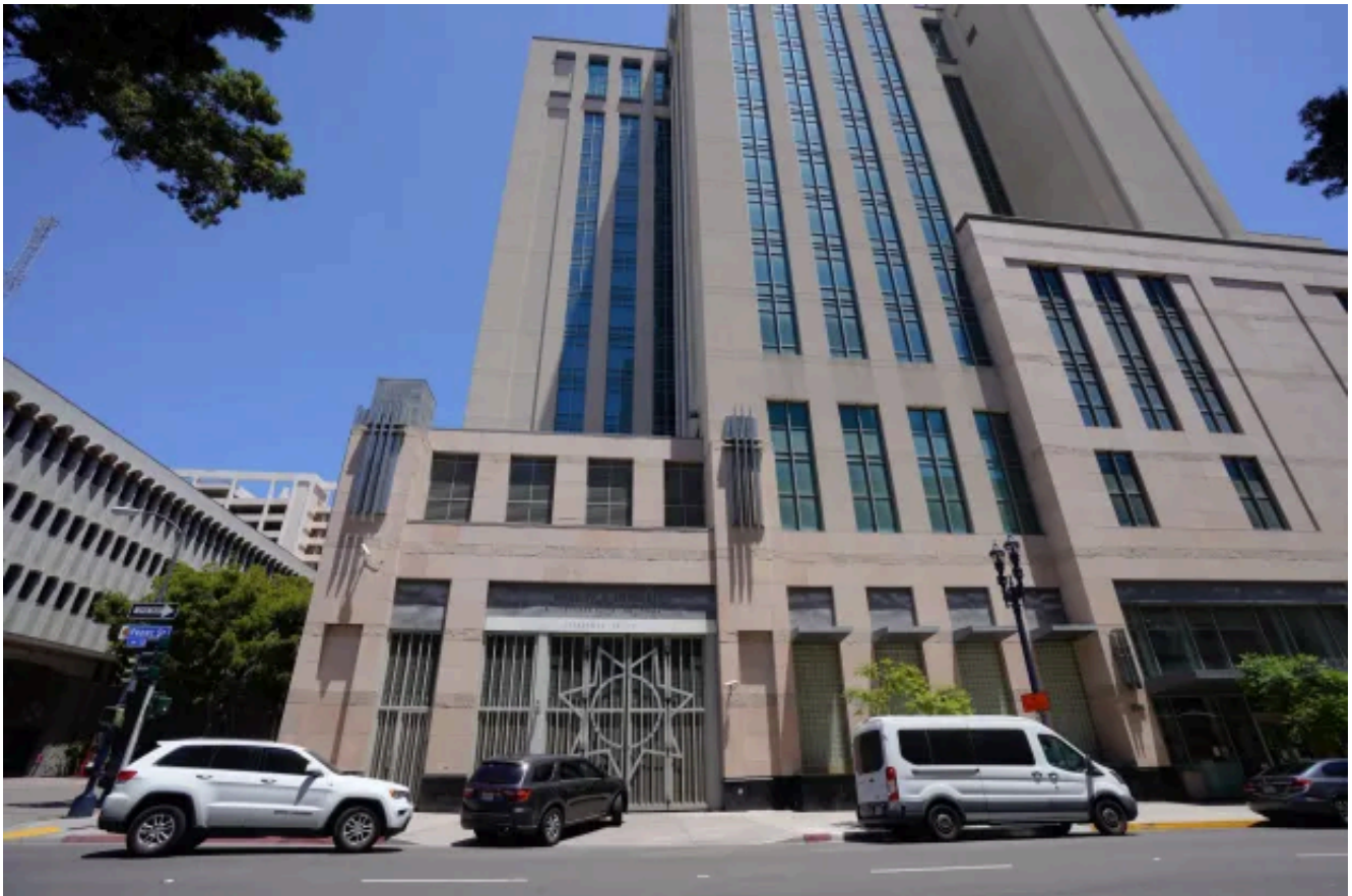
Entrance to the sheriff's intake at San Diego Central Jail in downtown San Diego. (Nelvin C. Cepeda / The San Diego Union-Tribune)
